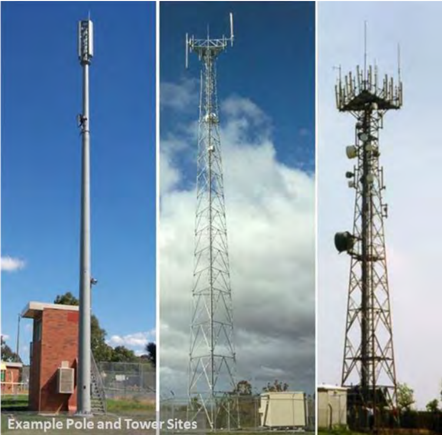
Figure 13 Example rooftop, pole and tower base stations
